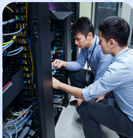
Optical cable construction and maintenance
